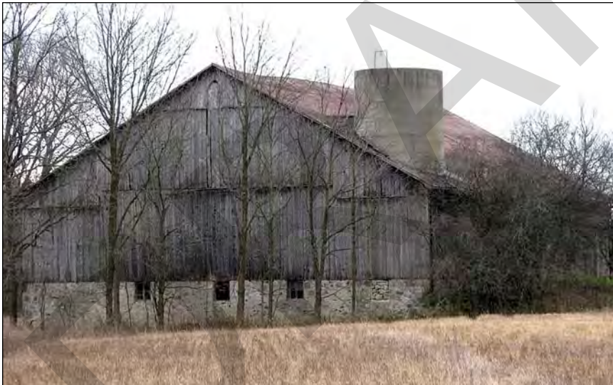
8. The property retains an expansive bank barn with a gable roof, a stone foundation and an unusual interior silo.
