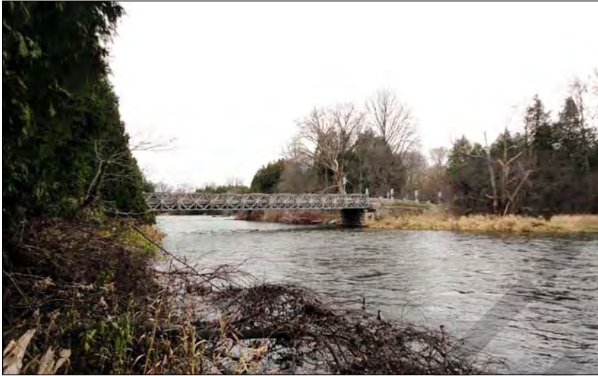
5. The Niska Road Bridge is set within a natural landscape characterized by woods and wetlands.
