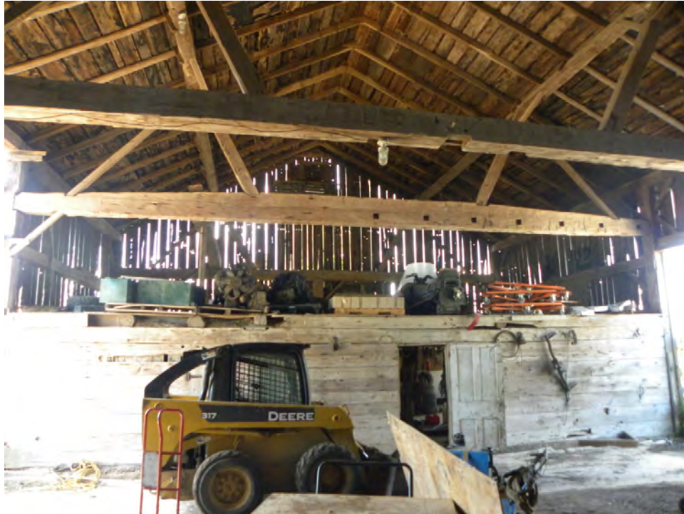
Plate 22: Looking towards east end of the barn. Horizontal beam in the rear is the swing beam. The beam is defined by its thickness, distinctive camber, and the square holes would have held joists.
