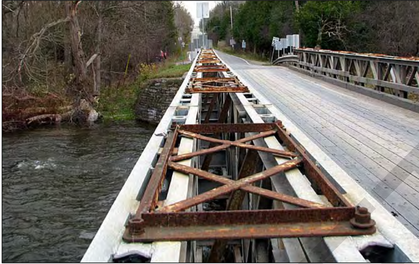
9. A bracing frame connects the top chords of the trusses.
