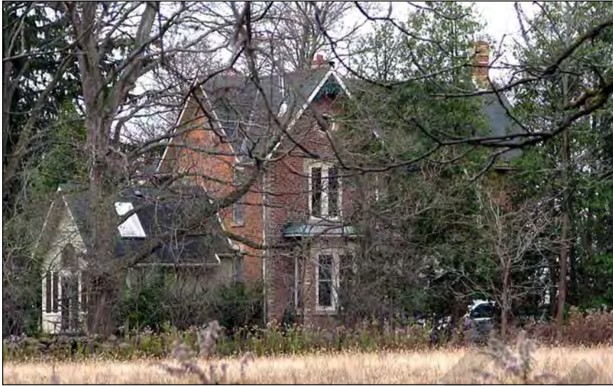
7. A late 19 th century farmhouse with dichromatic brickwork at 6769 Niska Road relates historically to the Buchanan Homestead.
