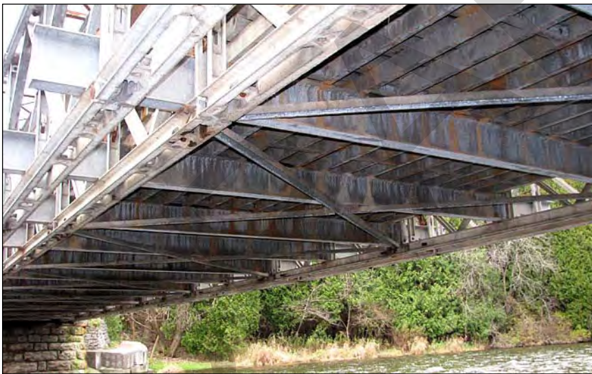
C-12. The deck assembly comprises transverse transoms (floor beams), longitudinal stringers and diagonal sway bracing. Two layers of timber decking are supported on the stringers.
