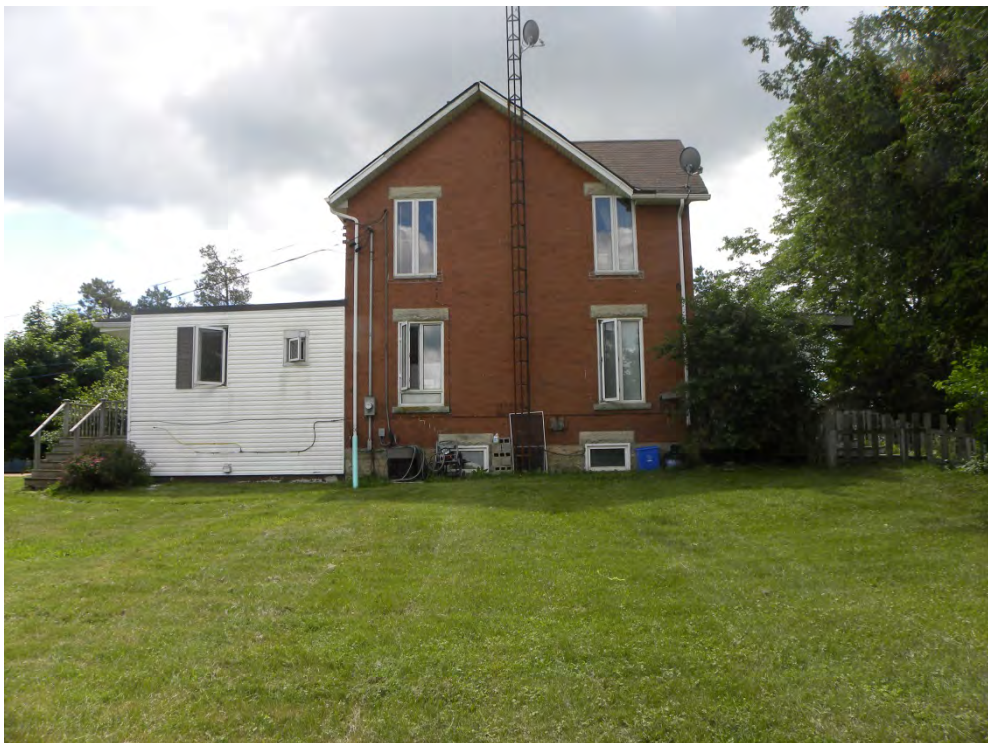
Plate 11: West façade of house showing stone foundation, brick construction, and rear addition. The window sills on the ground floor are constructed of stone, while the second floor sills have been replaced with concrete
