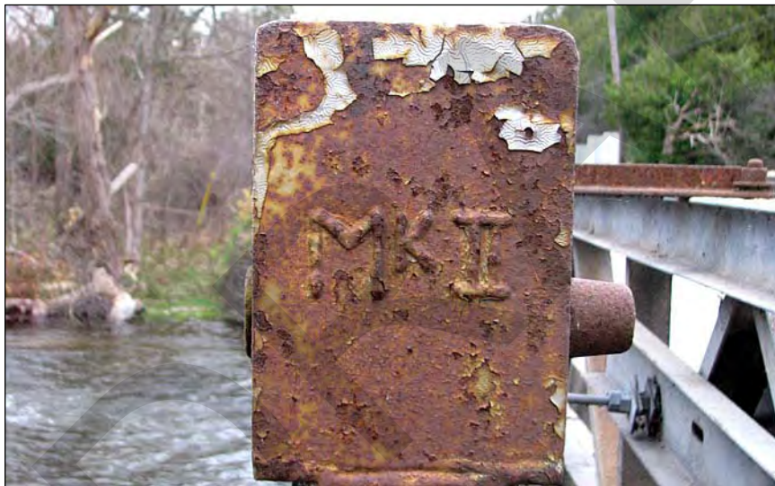
10. Some of the truss components are identified with standard Bailey bridge designations as exemplified by the 'Mk II' on the northwest end post.
