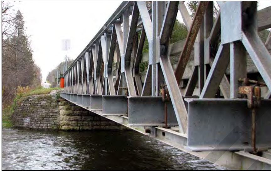
13. The transoms are supported on the bottom chords of the trusses.
