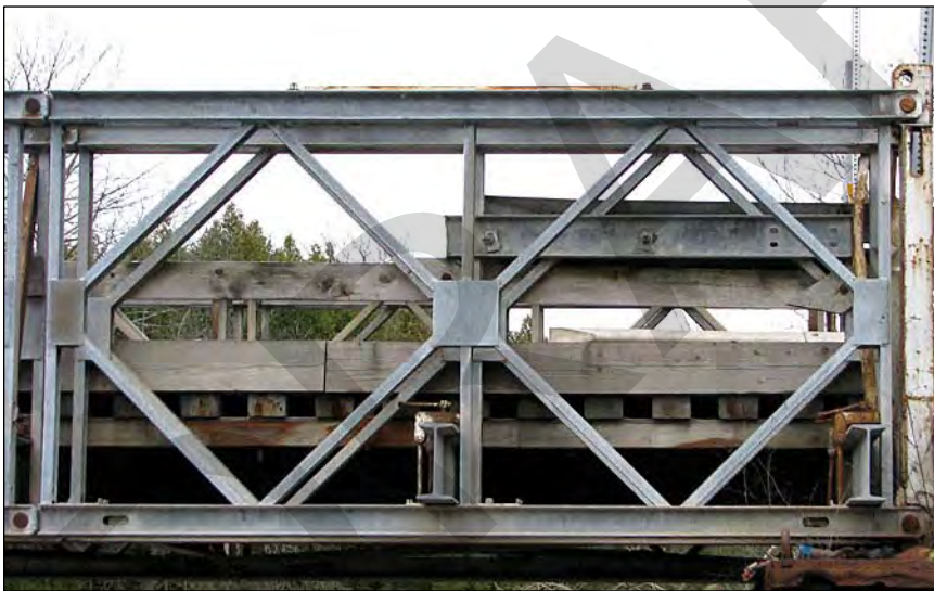
8. Each truss contains eight panels of the typical double diamond design that are 5-ft. 1-in. (1.55 m) high and 10-ft. 0-in. (3.05 m) long.
