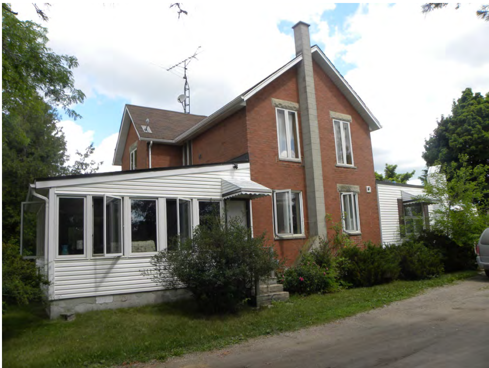
Plate 9: East façade of the house showing window arrangement, concrete chimney, and front and rear additions
