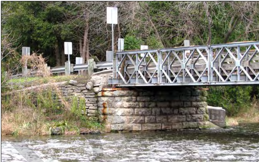
4. The east and west abutments are flanked by retaining walls to the north and south sides.
