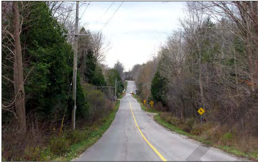
1. Niska Road follows a generally straight alignment down into the Speed River valley. A utility right-of-way parallels the south side of the roadway.
