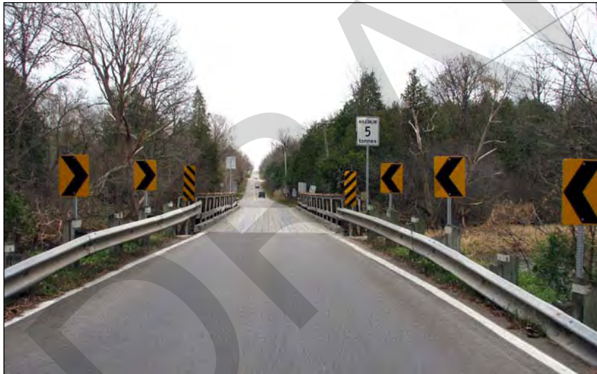
4. Chevron signs and guiderails funnel traffic from the two-lane roadway onto the one-lane bridge. The bridge has a 5 tonnes posted weight limit.
