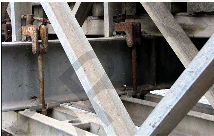
14. A detail of the deck assembly depicts the transom clamps that connect the transoms to the bottom chords.
