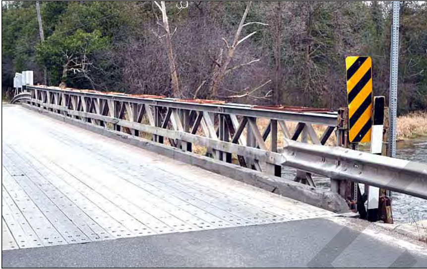
7. There are two galvanized trusses on each side of the bridge.
