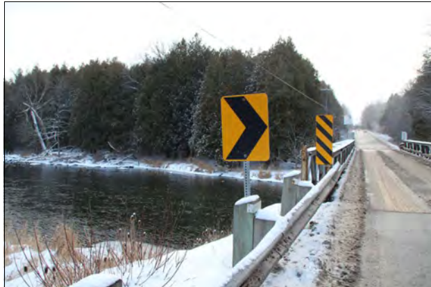
Figure 8 Niska Road bridge looking southwest
