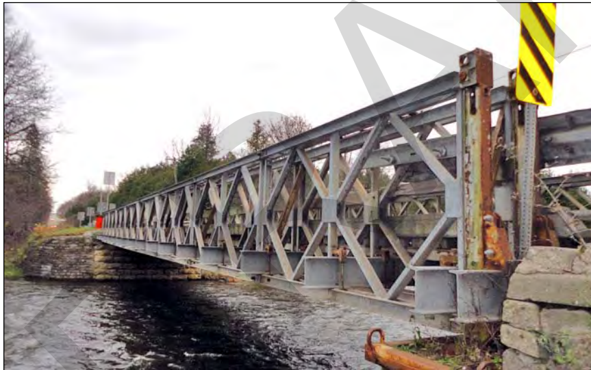
2. The one-span structure spans approximately 80-ft. (24 m) and features double truss, single storey Bailey panels.
