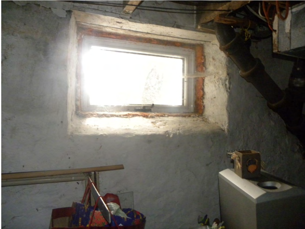
Plate 12: Basement wall showing parged stone finish, and modern vinyl window
