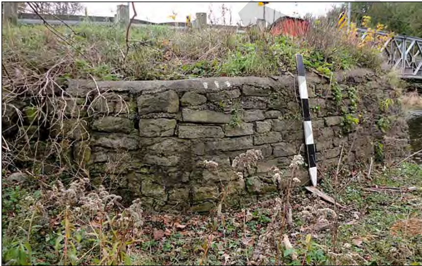
6. The retaining walls contain rubble concrete laid in a random pattern.
