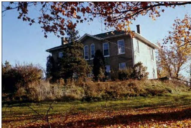
Figure 10 Lot 13, Con 5 Puslinch, Steele/Anderson House Gordon Couling 1973 - 00239 Wellington County Museum
