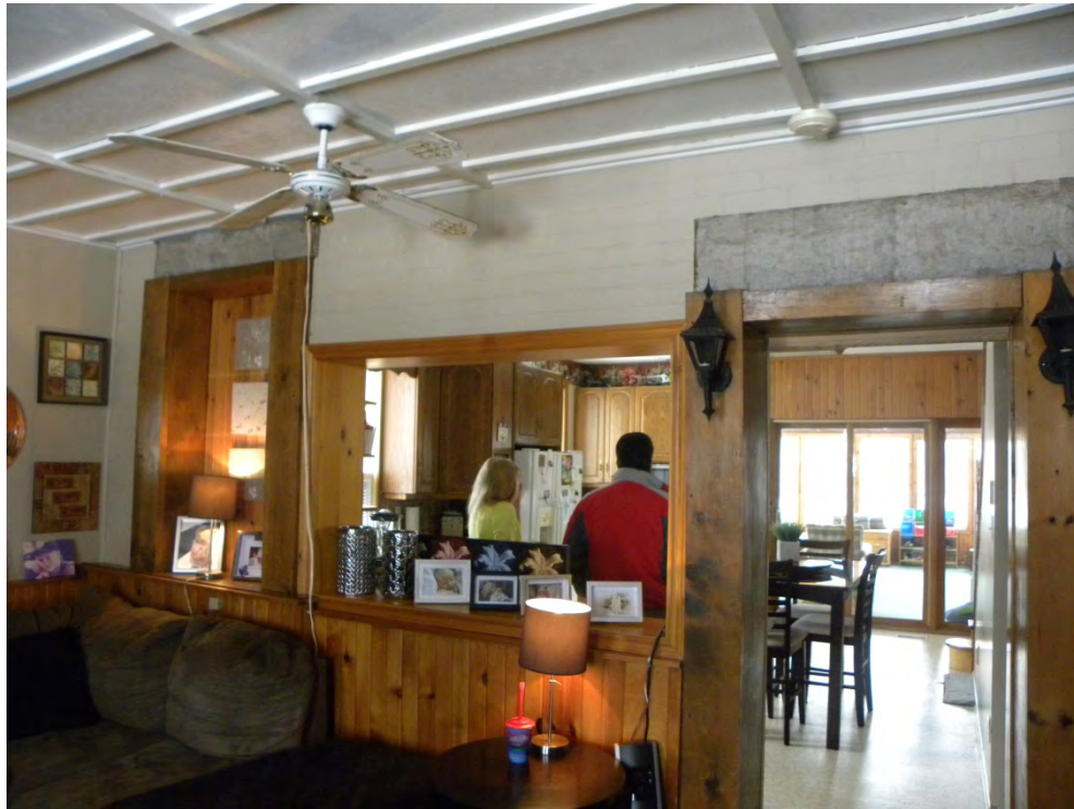
Plate 14: Interior of rear addition, looking south towards kitchen showing exposed brick wall and former exterior sills above door and window opening
