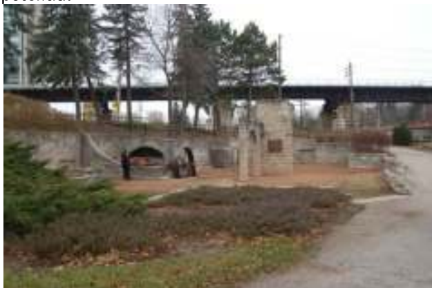
Plate 9: North view of the former Allan's Mill complex; Area retains potential for deeply buried archaeological resources and requires Stage 2 trenching if impacted by project design.
