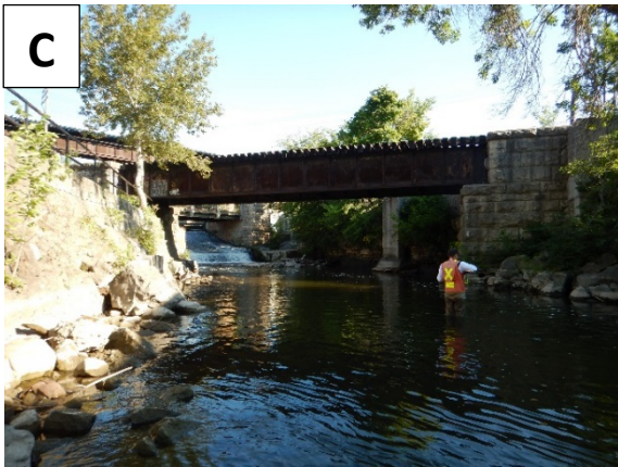
Looking upstream at the GJR railway bridge crossing.
