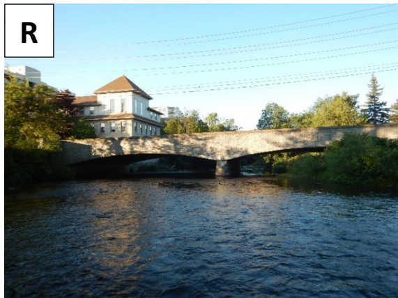
Looking downstream at the Neeve Street bridge crossing.
