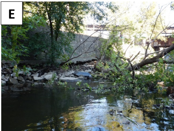
Recently fallen tree downstream of GJR railway bridge crossing (west bank).
