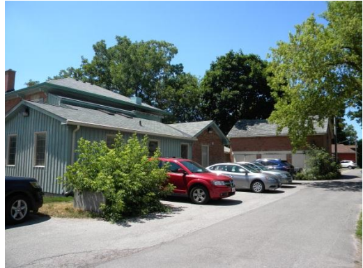
Figure 5 – Rear of house from laneway (2016).
