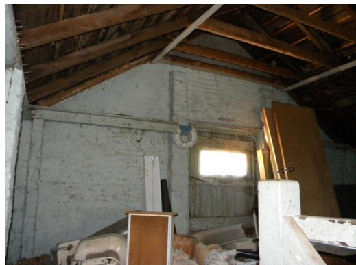
Figure 9 – Interior of upper gable wall showing brick construction method.
