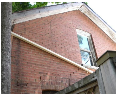
Figure 8 – Southwest gable wall (2016).
