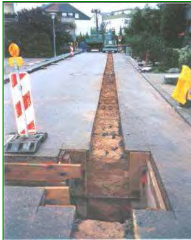
Figure 11.5 Laying District Heat Feeders in Mannheim
