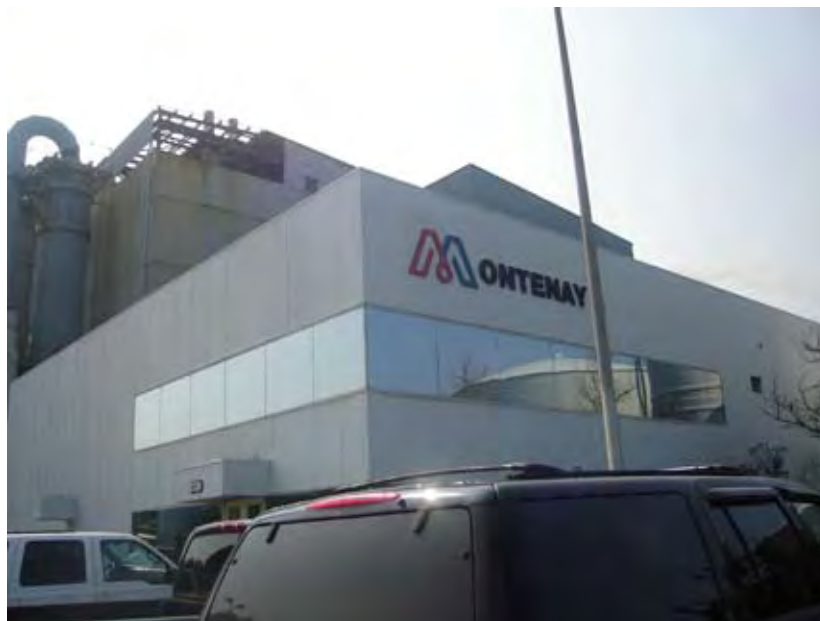
Figure 11.7 Modern Municipal Waste-to-Energy Plant
