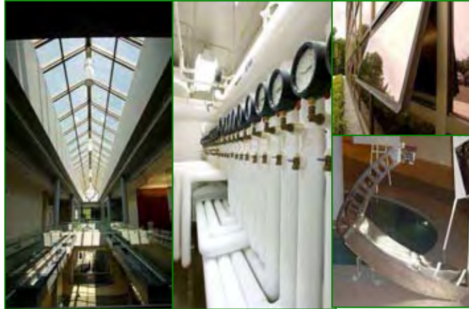
Figure 8.3 Guelph Hydro Administrative Centre Energy Efficient Features
