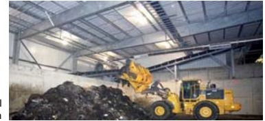
Galvanized steel roof system
