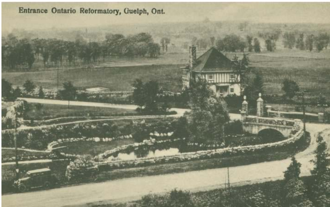
Photograph 4: 1920's Picture of Dry Stone Wing Wall with Circular End Treatment. The height of the wall is noticeably taller. The existing wall has been partially buried due to road grading. Photo from the Guelph Civic Museum.
