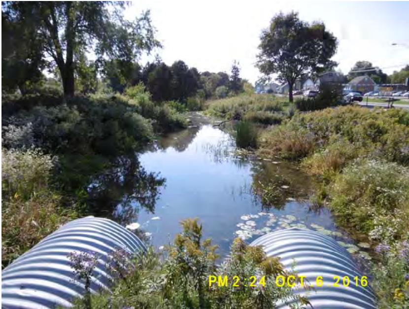
Downstream of twin CSP culverts
