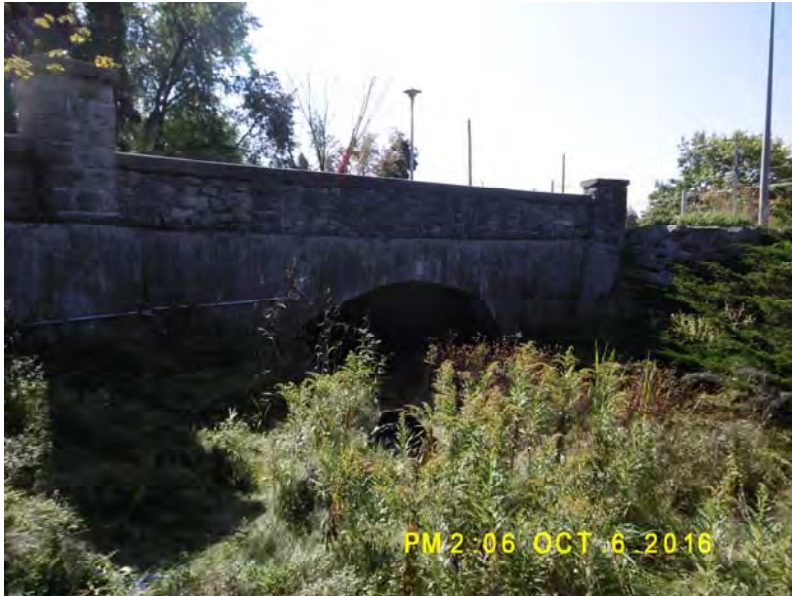
Former Reformatory driveway crossing
