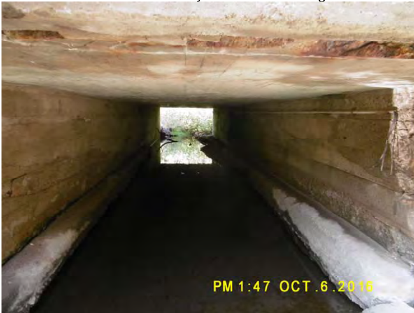
Clythe Creek culvert
