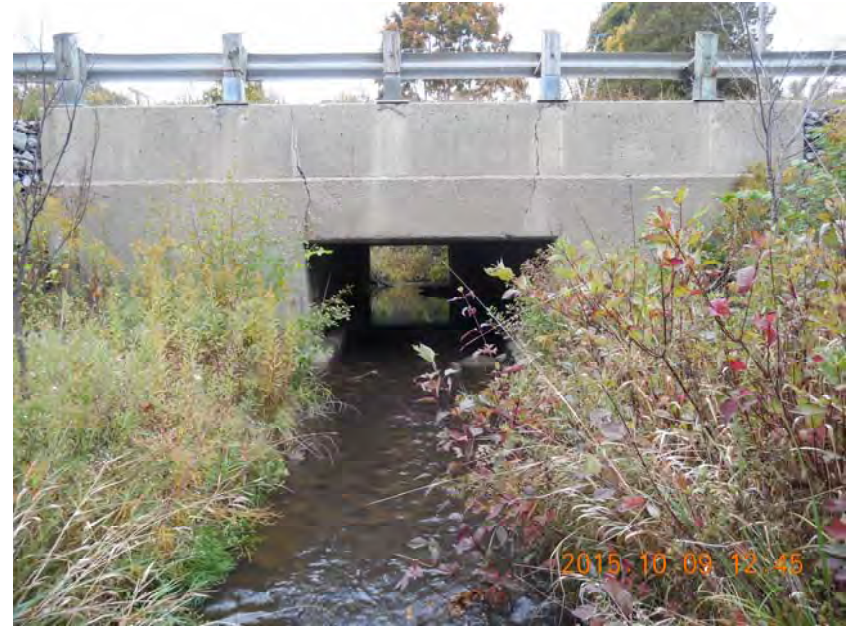
Downstream face of Clythe Creek
