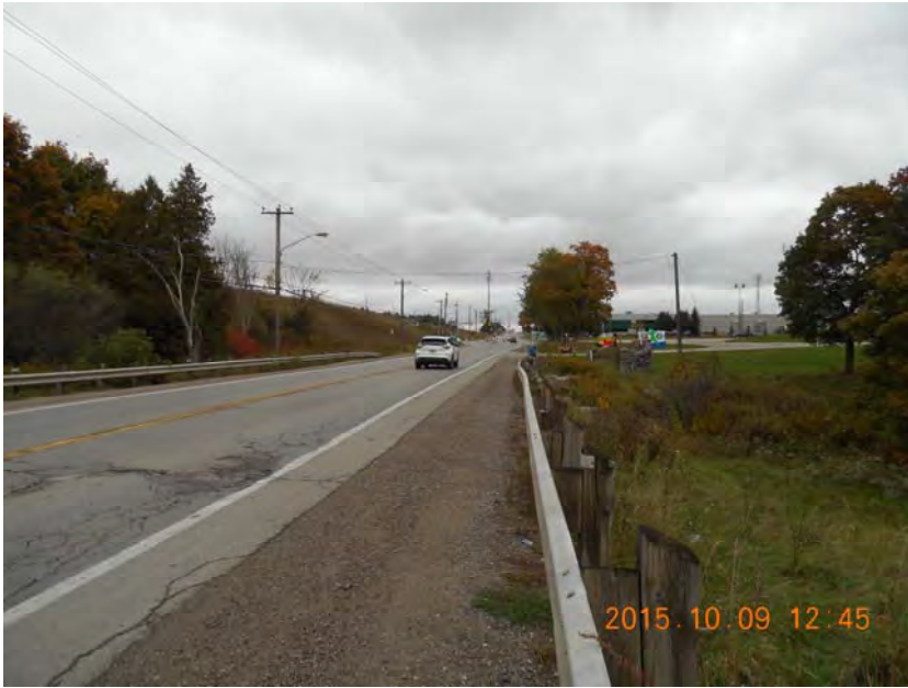
York Road at Clythe Creek crossing
