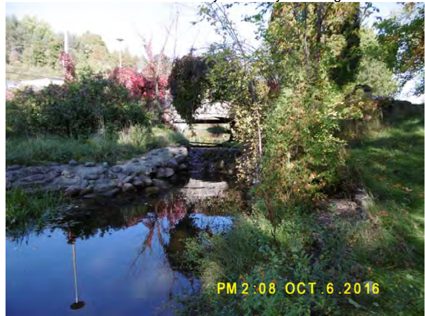
Lined channel downstream of former Reformatory driveway
