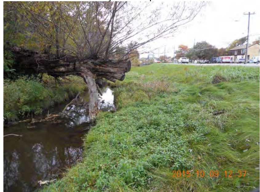
Creek in close proximity to the roadway
