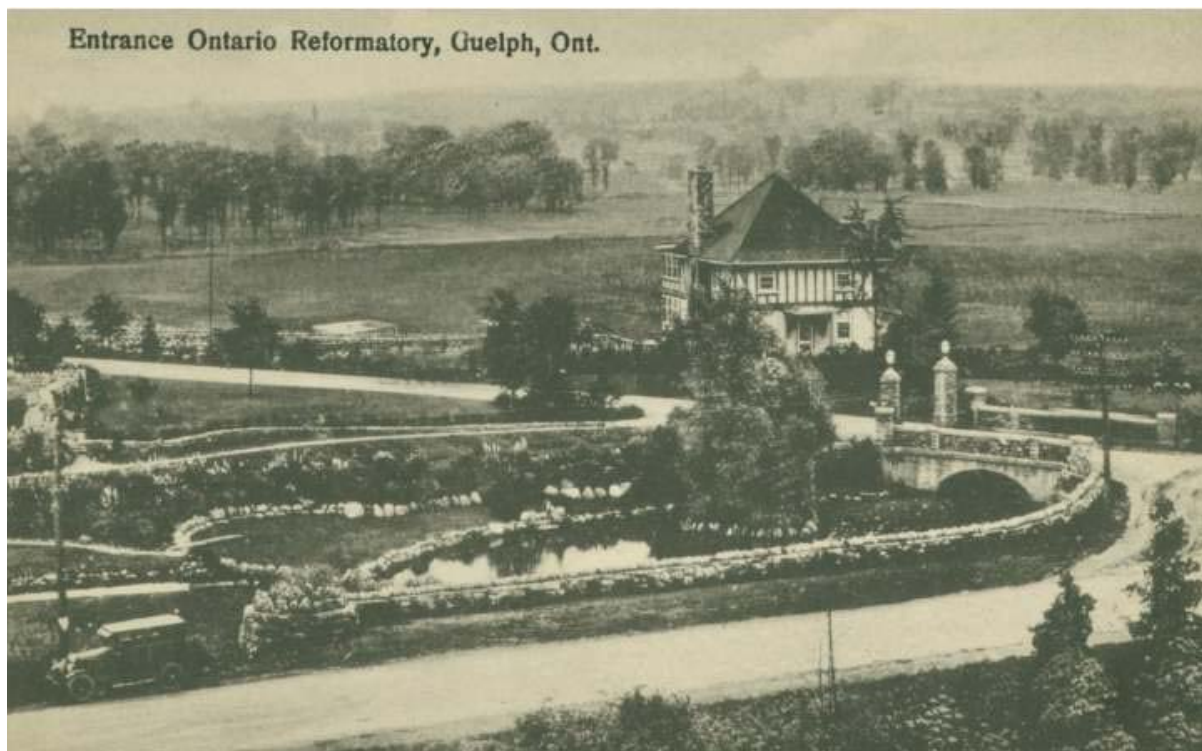
Photograph 5A: 1920 picture of dry stone wing wall with circular end treatment. The height of the wall is noticeably taller. The existing wall has been partially buried due to road grading.
