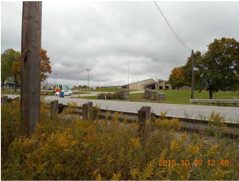
York Road east of Clythe Creek crossing
