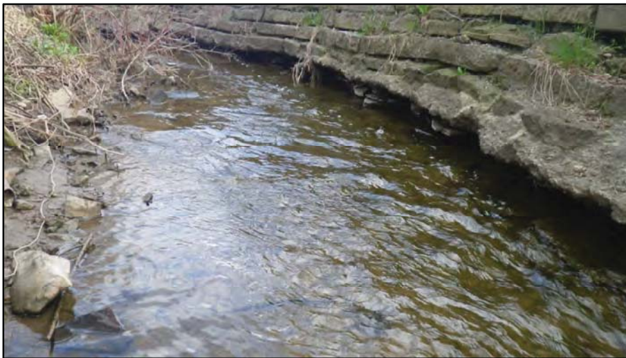
24. Reach HC-1: Concrete block wall at channel bend is undermined.
