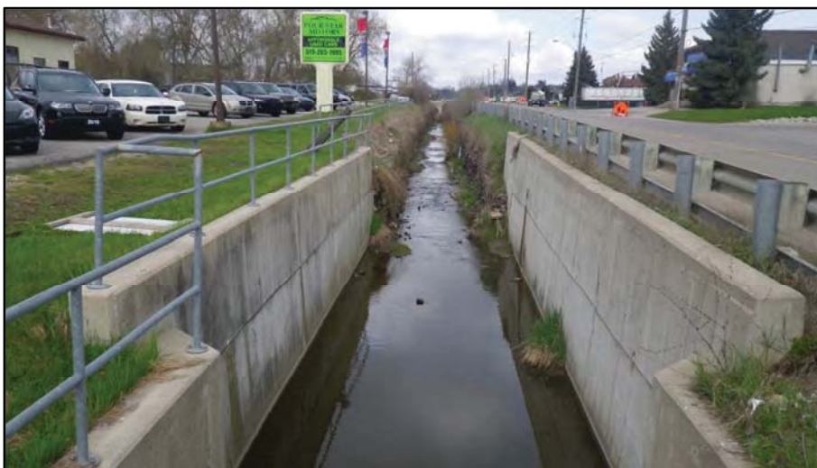
28. Reach HC-1: Looking upstream from Beaumont Cres crossing. Channel is lined with concrete for approximately 18 m.
