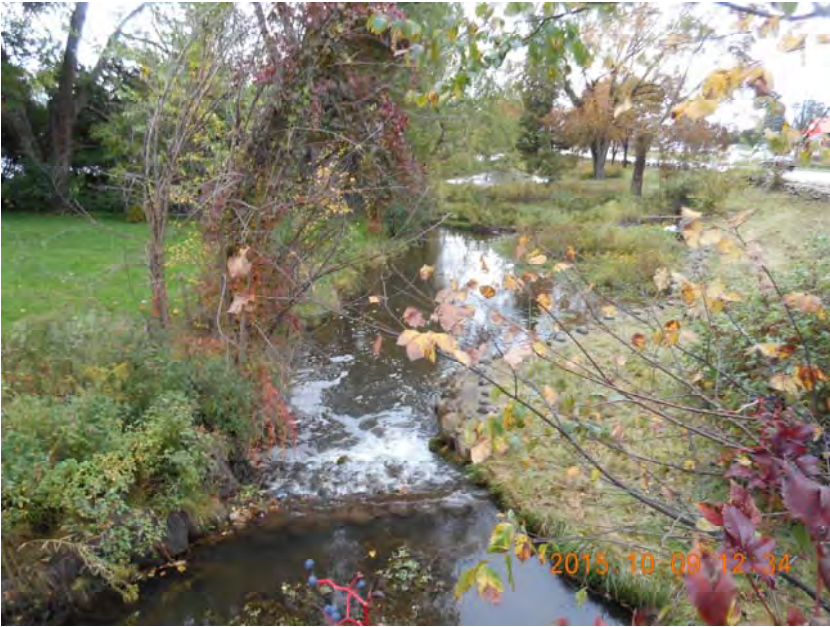
Drop structure downstream of former Reformatory driveway crossing
