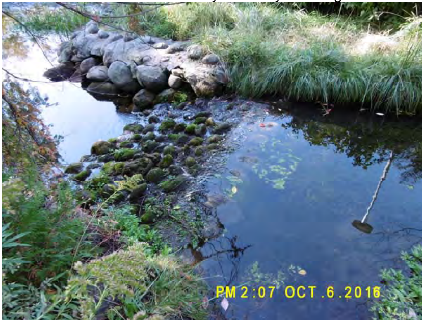
Downstream of former Reformatory driveway crossing Note drop structure
