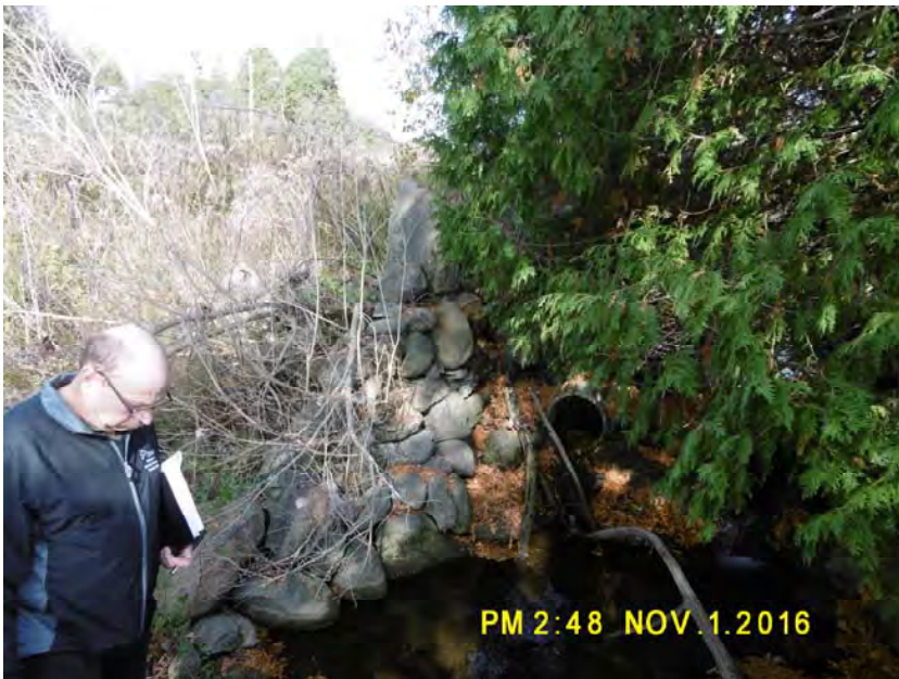
Cultural heritage drop structure with side walls and pipes
