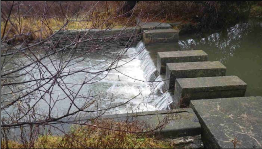
15. Flow control structure downstream from Hadati Creek confluence.
