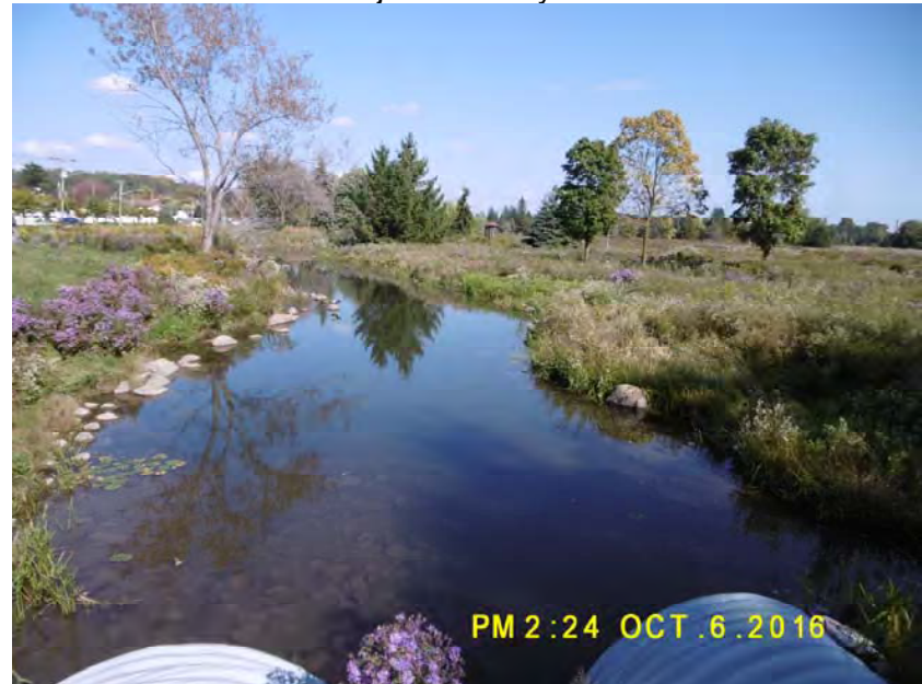
Upstream of twin CSP crossing into park parking lot
