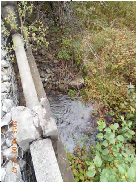
Upstream face of Clythe Creek crossing
