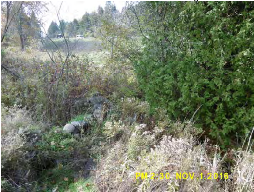
Cultural heritage wall close to York Road culvert
