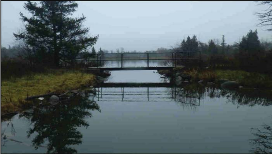
11. Looking upstream along the North Pond connection channel and pedestrian bridge.
