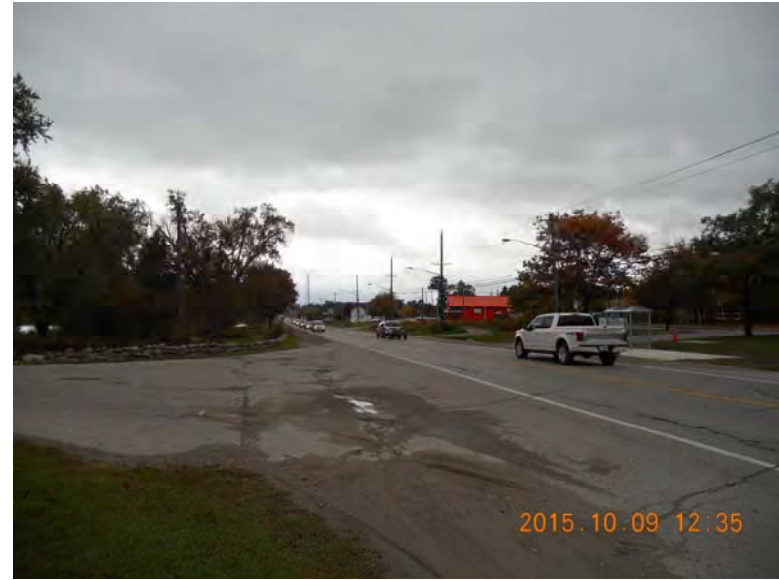
Former Reformatory driveway
