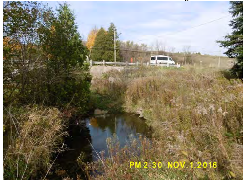
Pool feature immediately downstream of culvert
