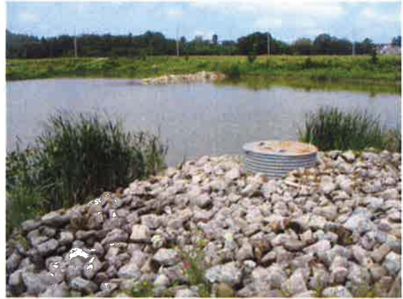
Photo 8: Storm water management pond collects runoff from the developing portion of the watershed near Starwood Drive and Grange Road. The pond discharges to the Creek just upstream of Watson Parkway (Site 5).
