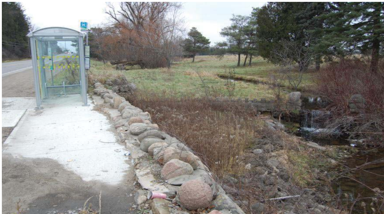
Photograph 1A: East side of entrance bridge. Only top of wall is visible
