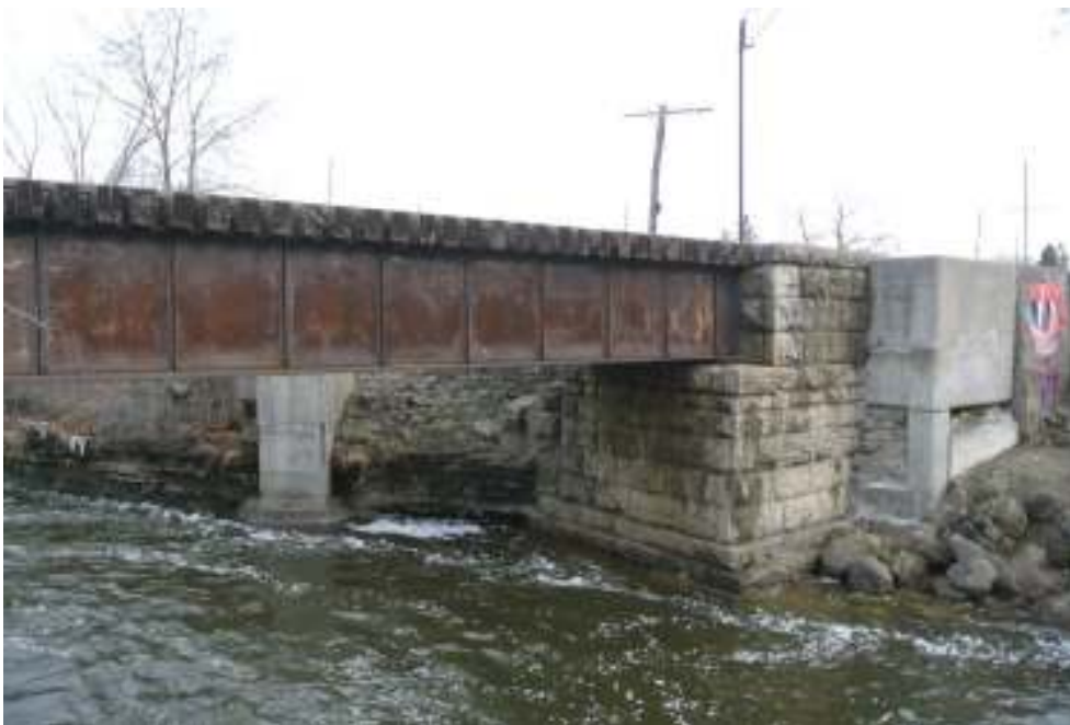
Plate 6: View northeast toward the east abutment of the bridge.
