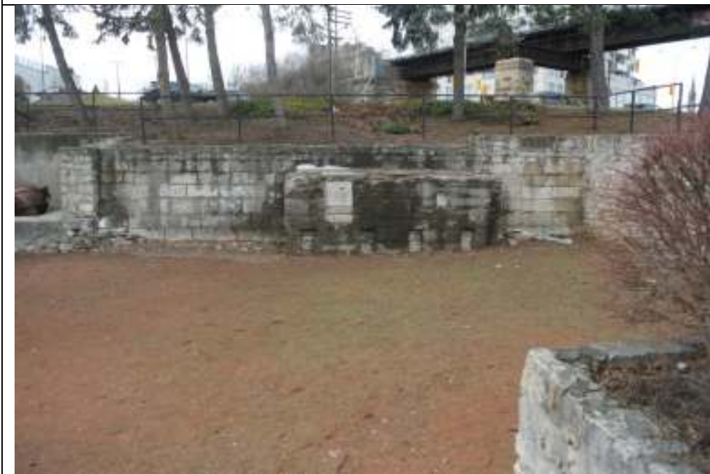
Plate 18: Detail the foundations on the west side of the property.
