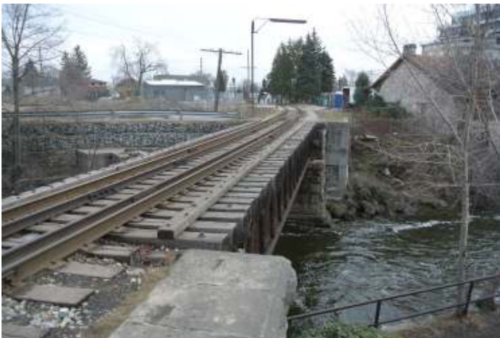
Plate 2: Oblique view of the bridge's south elevation, looking east.
