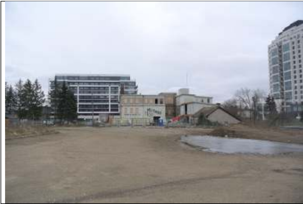
Plate 9: View south into the property from the north.
