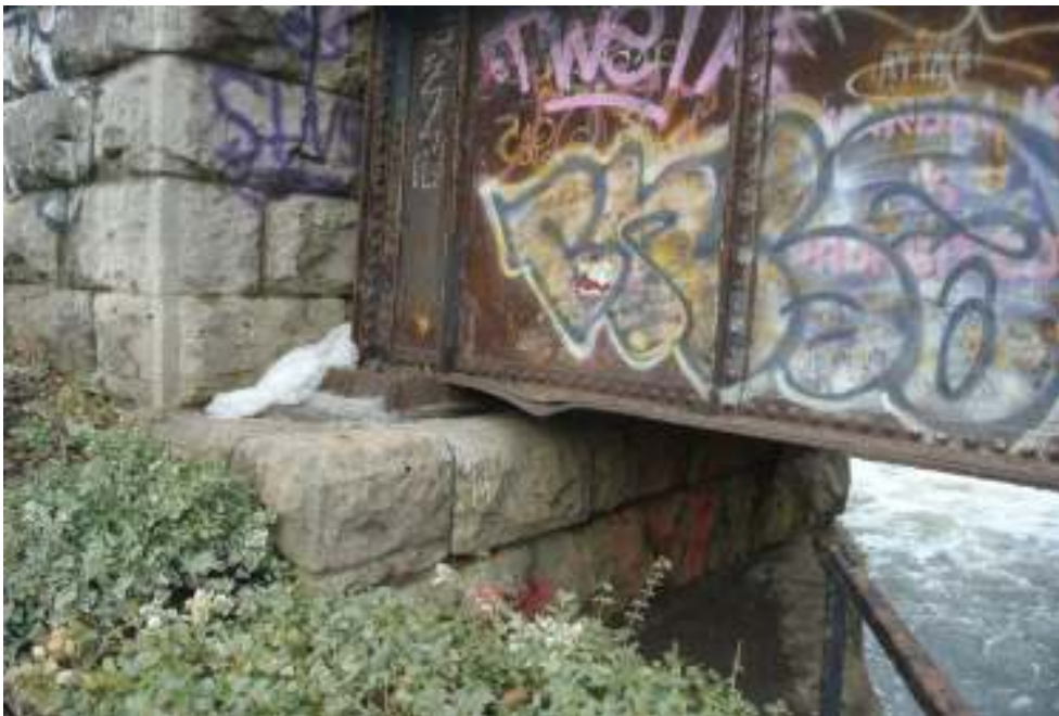
Plate 8: Detail of the bearings located on the west abutment.
