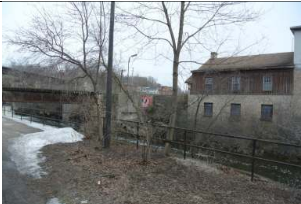
Plate 14: View of toward the Wellington Street Rail Bridge and 5 Arthur Street South, looking northeast.
