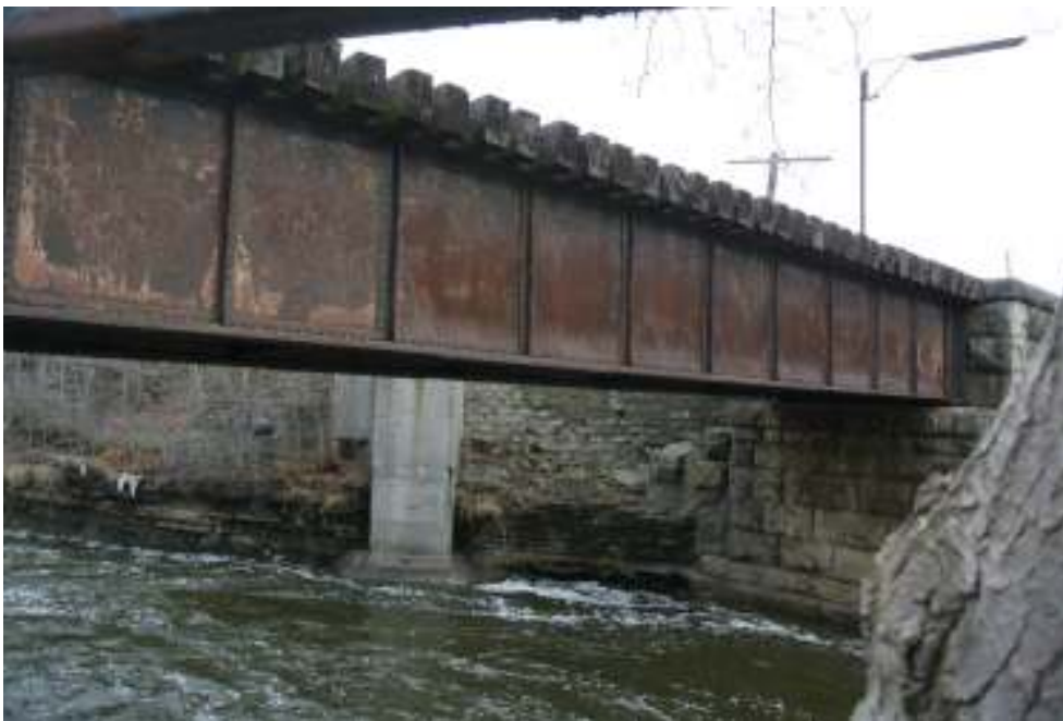
Plate 10: View of the plate-girder deck supporting the wood deck.
