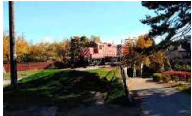
Plate 6: The Wellington Street Railway Bridge, looking east from the former Allan's Mills.
