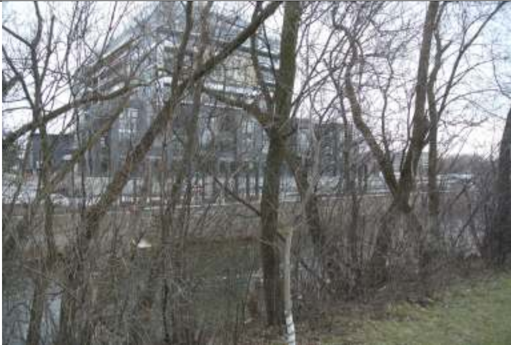
Plate 25: View west to the Speed River and 5 Arthur Street.
