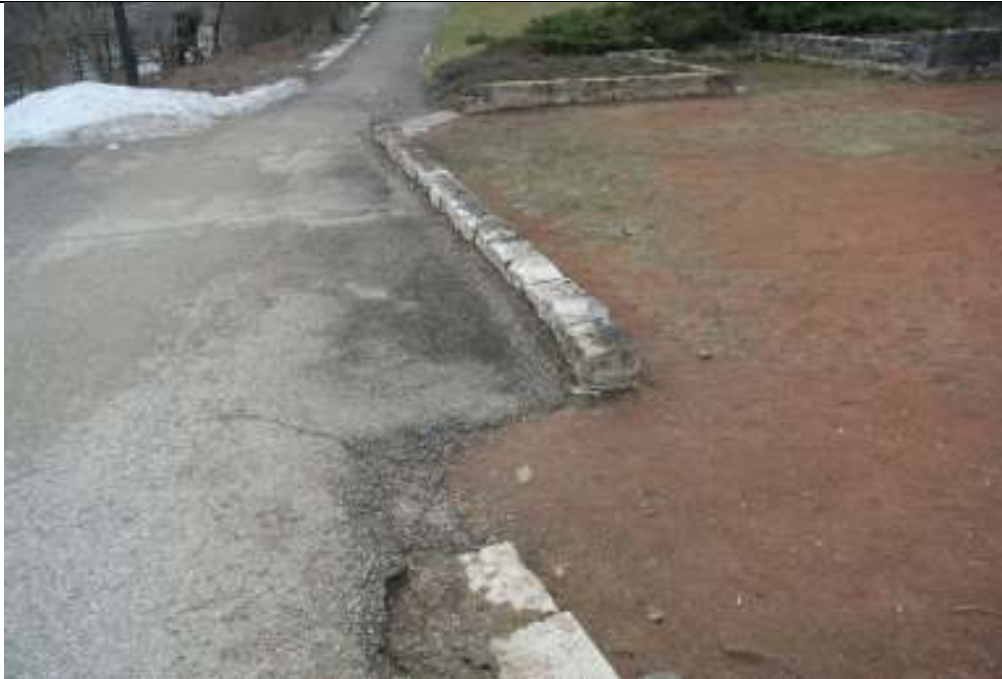
Plate 19: Detail of the former foundations at the east side of the ruins.
