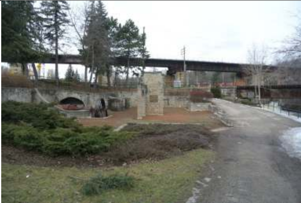
Plate 15: View of the Allan's Mill ruins, looking north.
