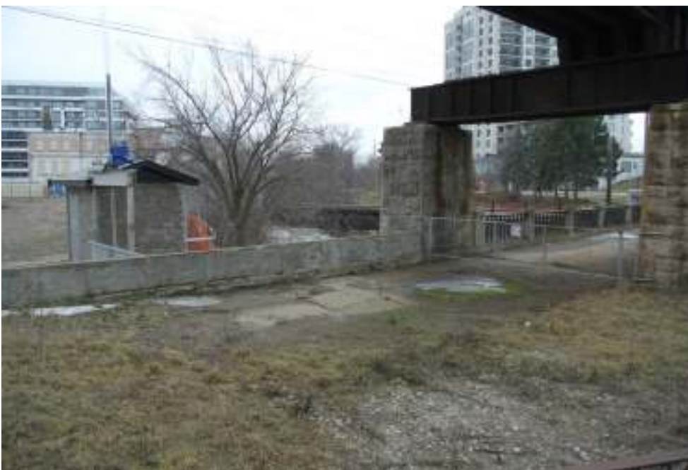
Plate 4: View south to the subject bridge with the former Allan's Bridge and portion's of the MacDonell Rail Viaduct in the foreground.
