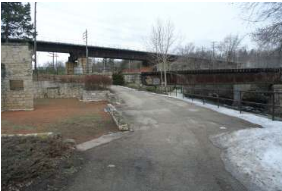
Plate 14: View north to Wellington Street Rail Bridge with Allan's Mill Ruins in foreground.
