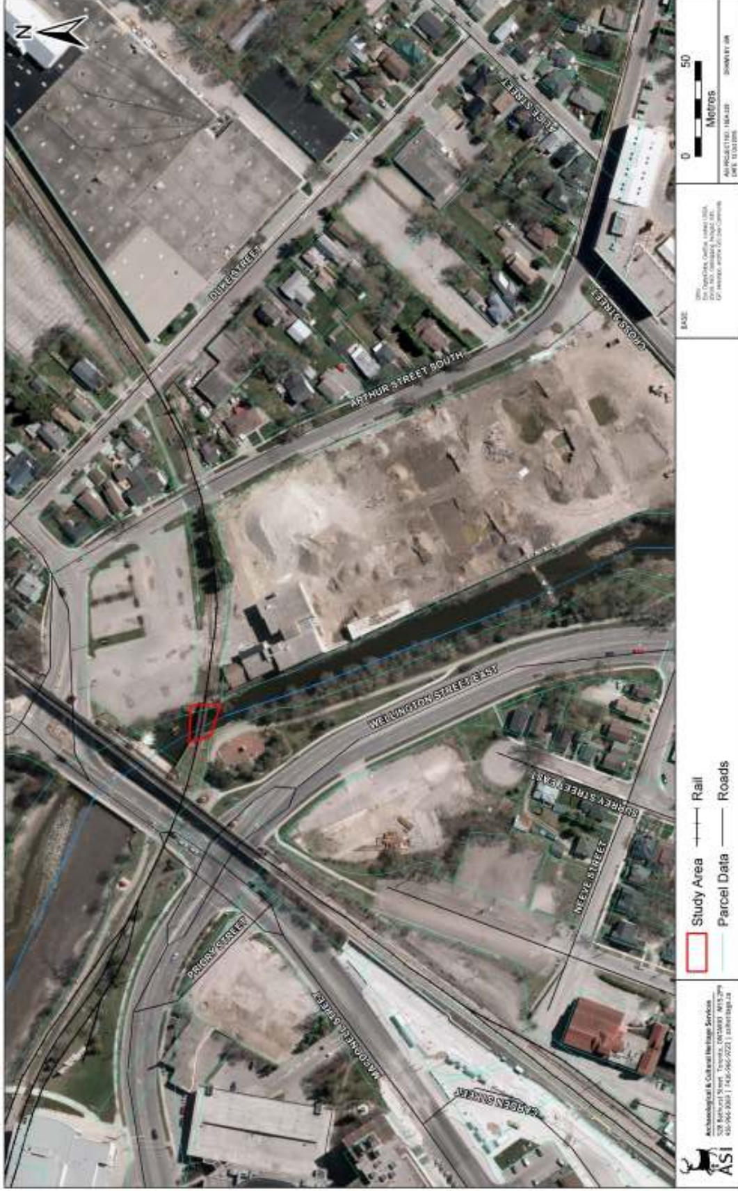
Figure 9: Orthographic image of the subject bridge
