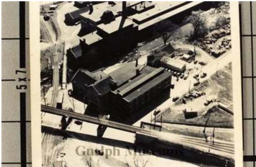
Figure 8: Aerial photograph of the subject bridge, c 1948.
