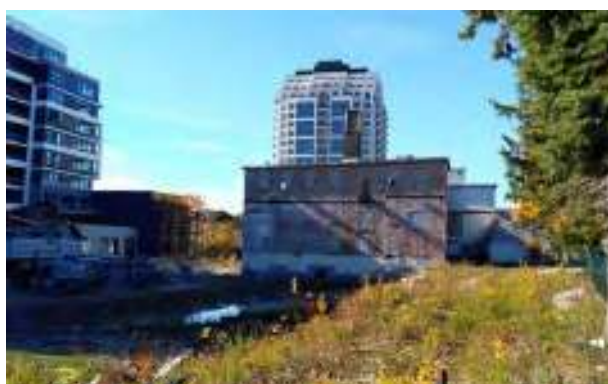
Plate 10: View west into the former Taylor-Forbes Mills property from Arthur Street.
