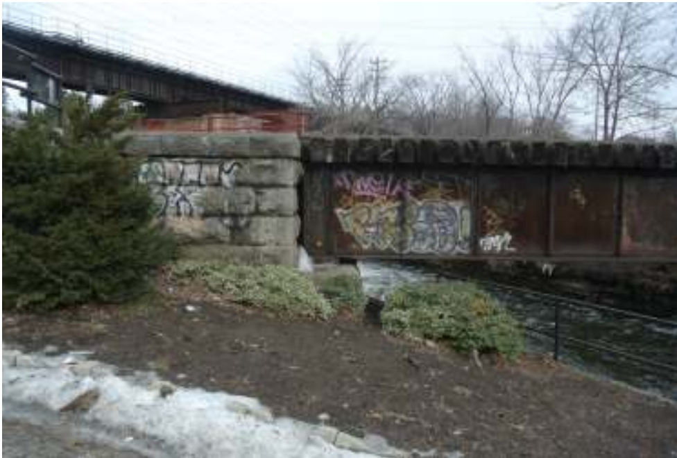
Plate 7: View north to the west abutment.
