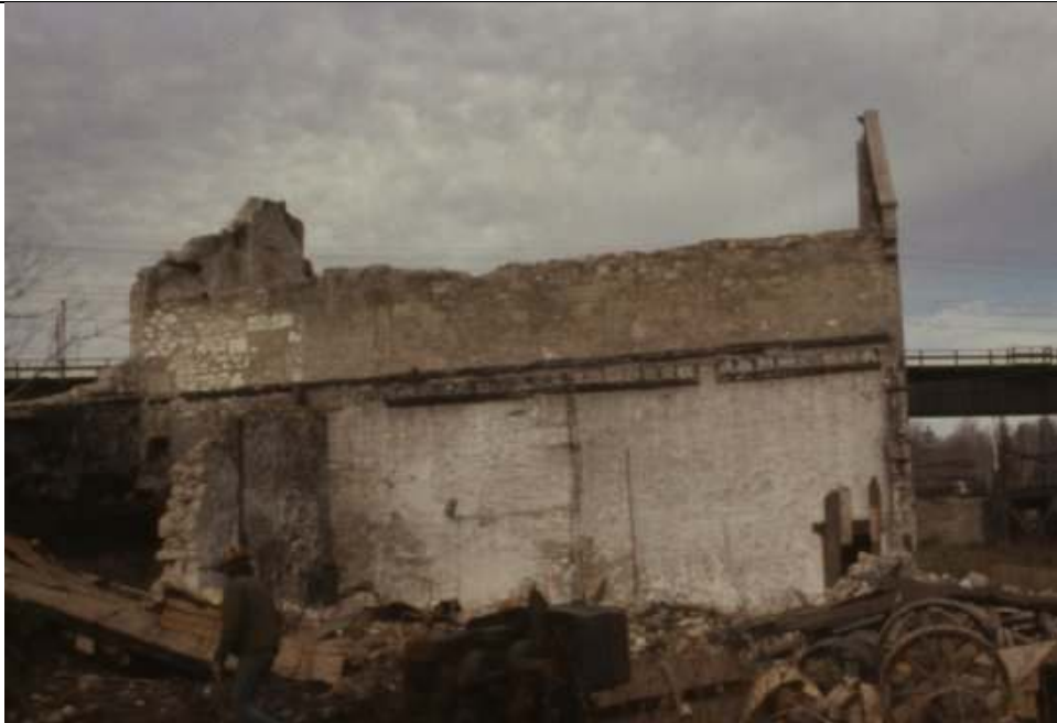
Plate 9: Demolition of Allan's Mill, November 10, 1975, Guelph Museums, Cat. No. 2009.32.754
