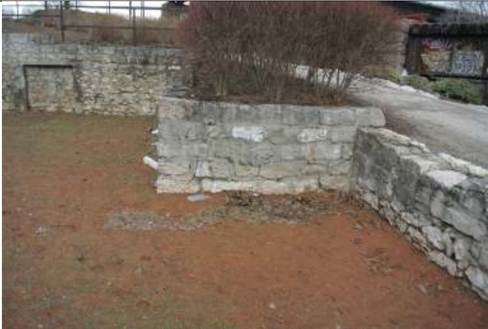
Plate 21: Detail of the former foundations.
