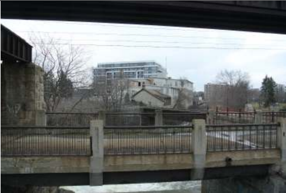
Plate 8: View south from underneath the MacDonell Street Rail Viaduct.
