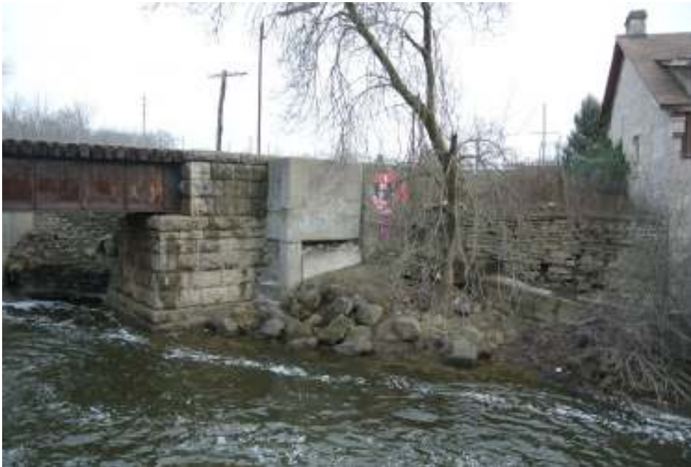
Plate 5: View northeast across the Speed River toward the east abutment of the subject bridge. Note the concrete stabilizing the original stone abutment.
