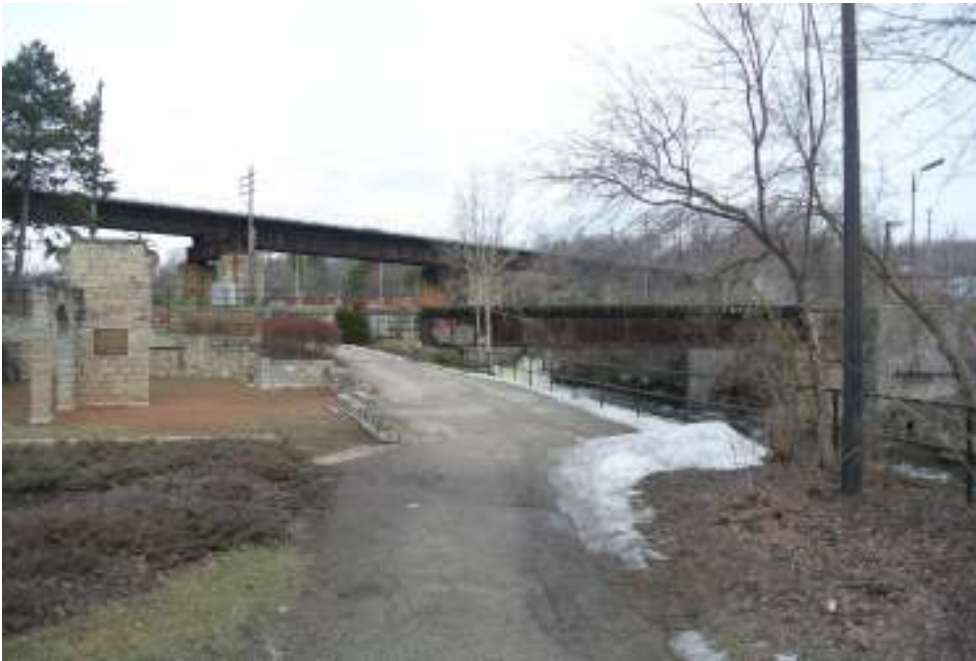
Plate 1: View toward the subject bridge from the south.
