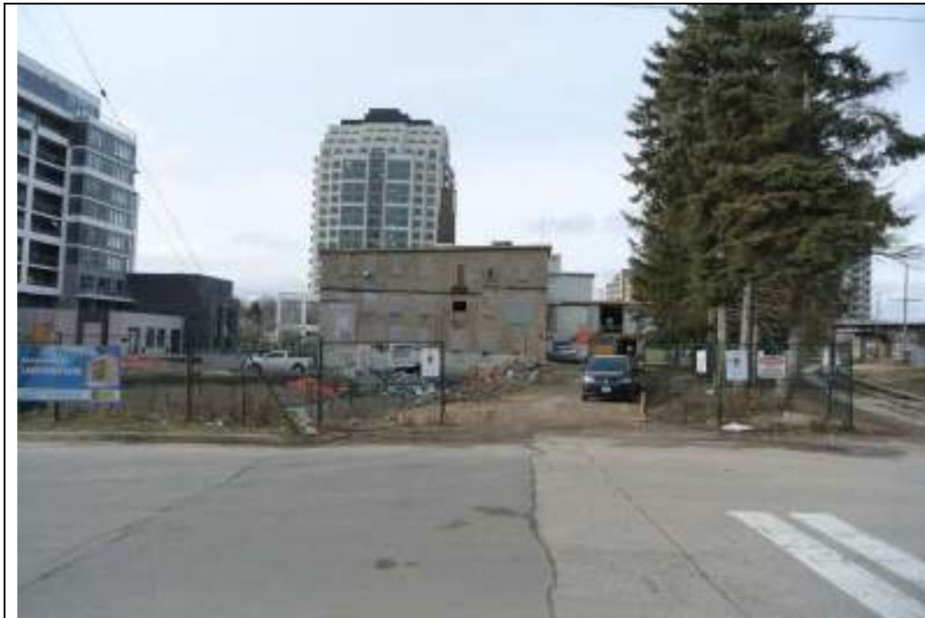
Plate 3: View west into the property from Arthur Street. Note buildings 2-5 in the foreground.
