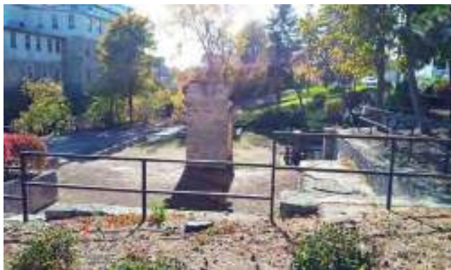
Plate 3: The former Allan's Mills (CHL 1), looking south.
