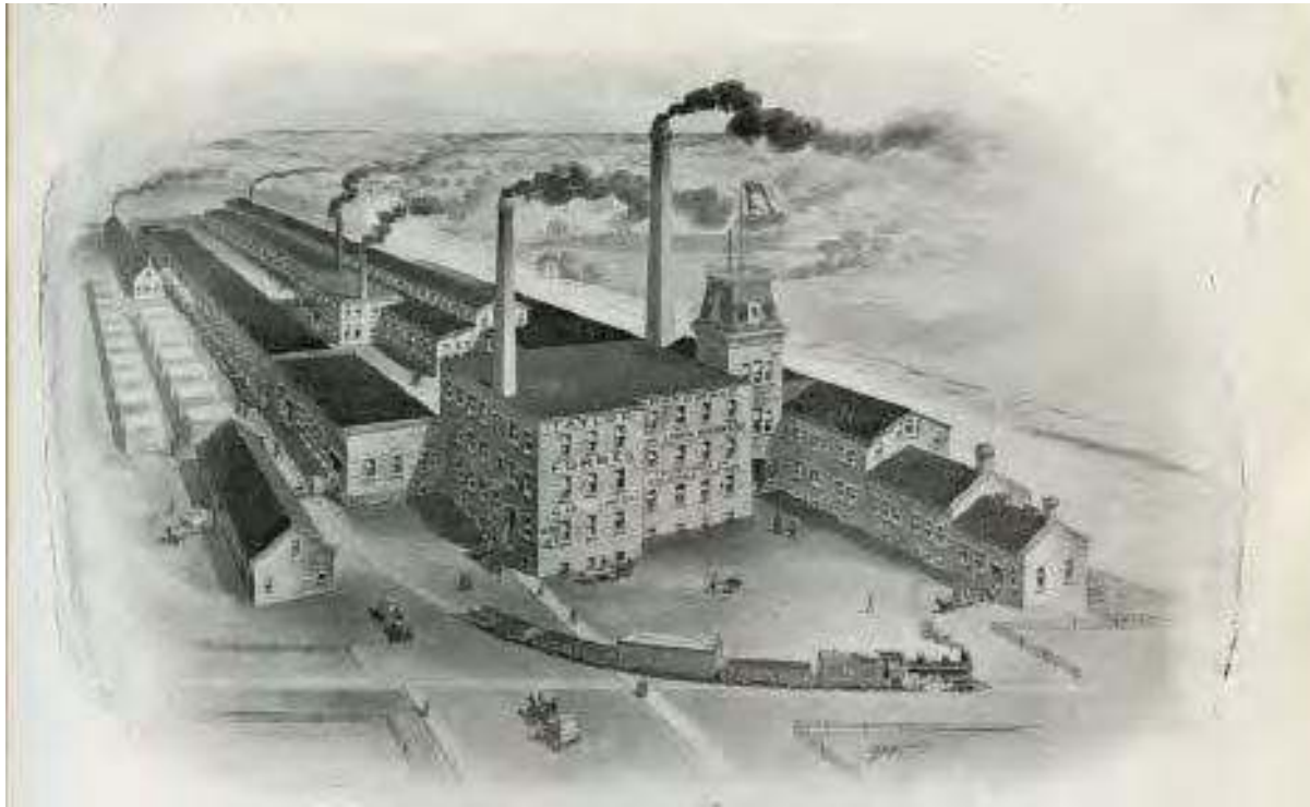
Figure 6: The Taylor-Forbes Mills, looking generally south
