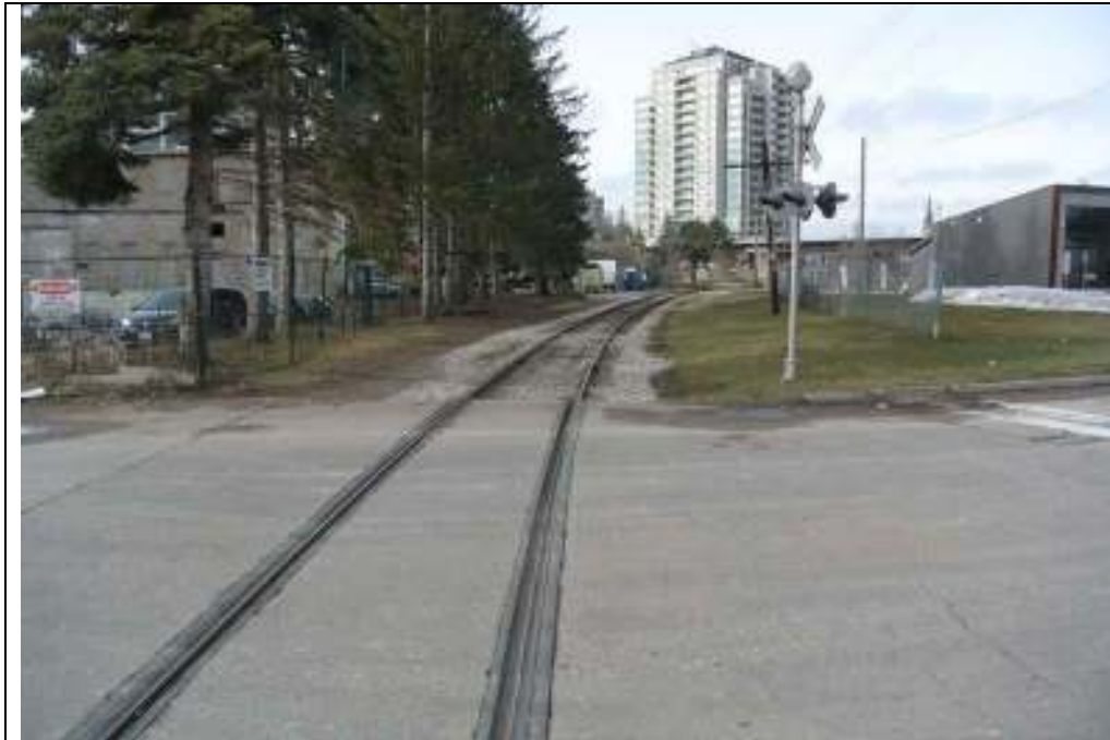
Plate 1: View west along the GJR tracks into the property.
