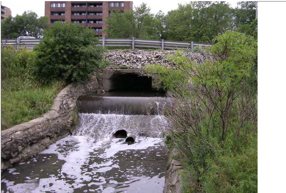
Photo 2: Barrier to upstream fish movement in Reach 1. July 27, 2005.
