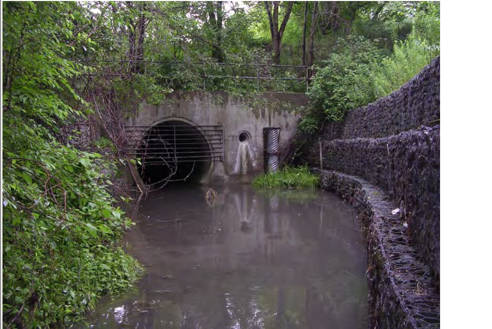
Photo 9: The origin of the watercourse is a storm sewer. July 27, 2005.
