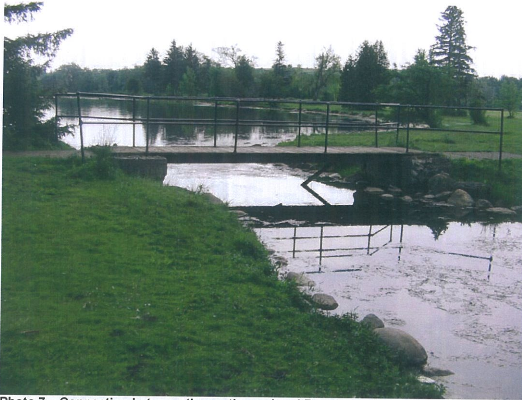
Photo 7 – Connection between the north pond and Reach 3 of Clythe Creek
