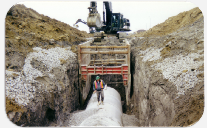
Typical Open-Cut Sewer Trench
