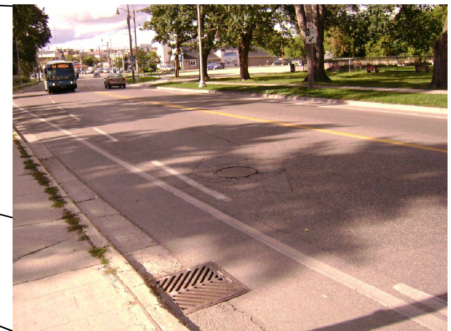
EXISTING YORK TRUNK SEWER ALIGNMENT AT GORDON STREET UNDERCROSSING
