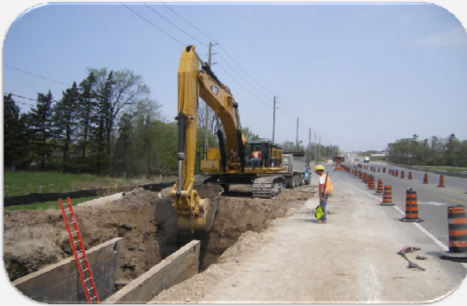
Open-Cut Sewer Construction on a Road Shoulder
