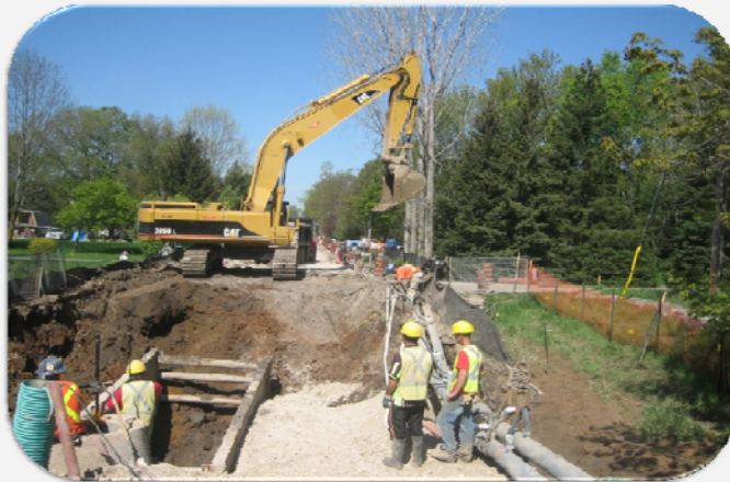
Typical Construction Crew
