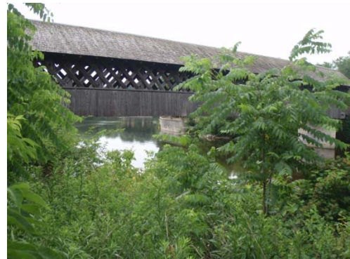
Town Lattice Covered Bridge
