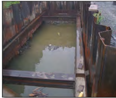
2. Water Flow is Diverted Across the Channel, Excavation is Pumped Out
