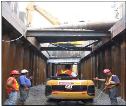
2. Water Flow is Diverted Across the Channel, Excavation is Pumped Out
