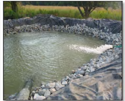
2. Water Flow is Diverted Across the Channel, Excavation is Pumped Out
