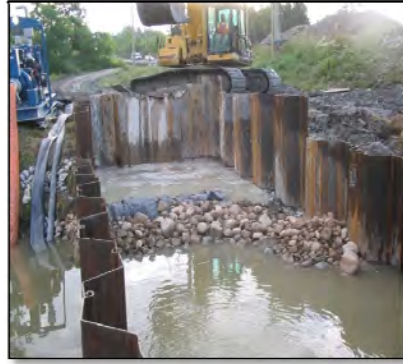
1. Sheet Piling is Installed Across the River
