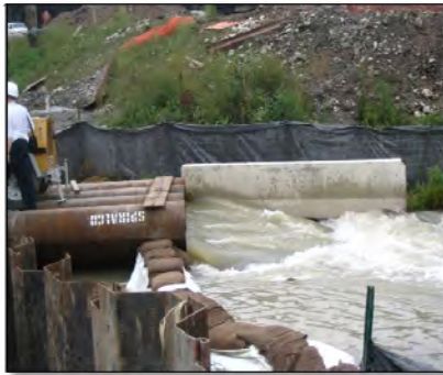
2. Water Flow is Diverted Across the Channel, Excavation is Pumped Out
