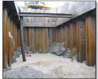
2. Water Flow is Diverted Across the Channel, Excavation is Pumped Out
