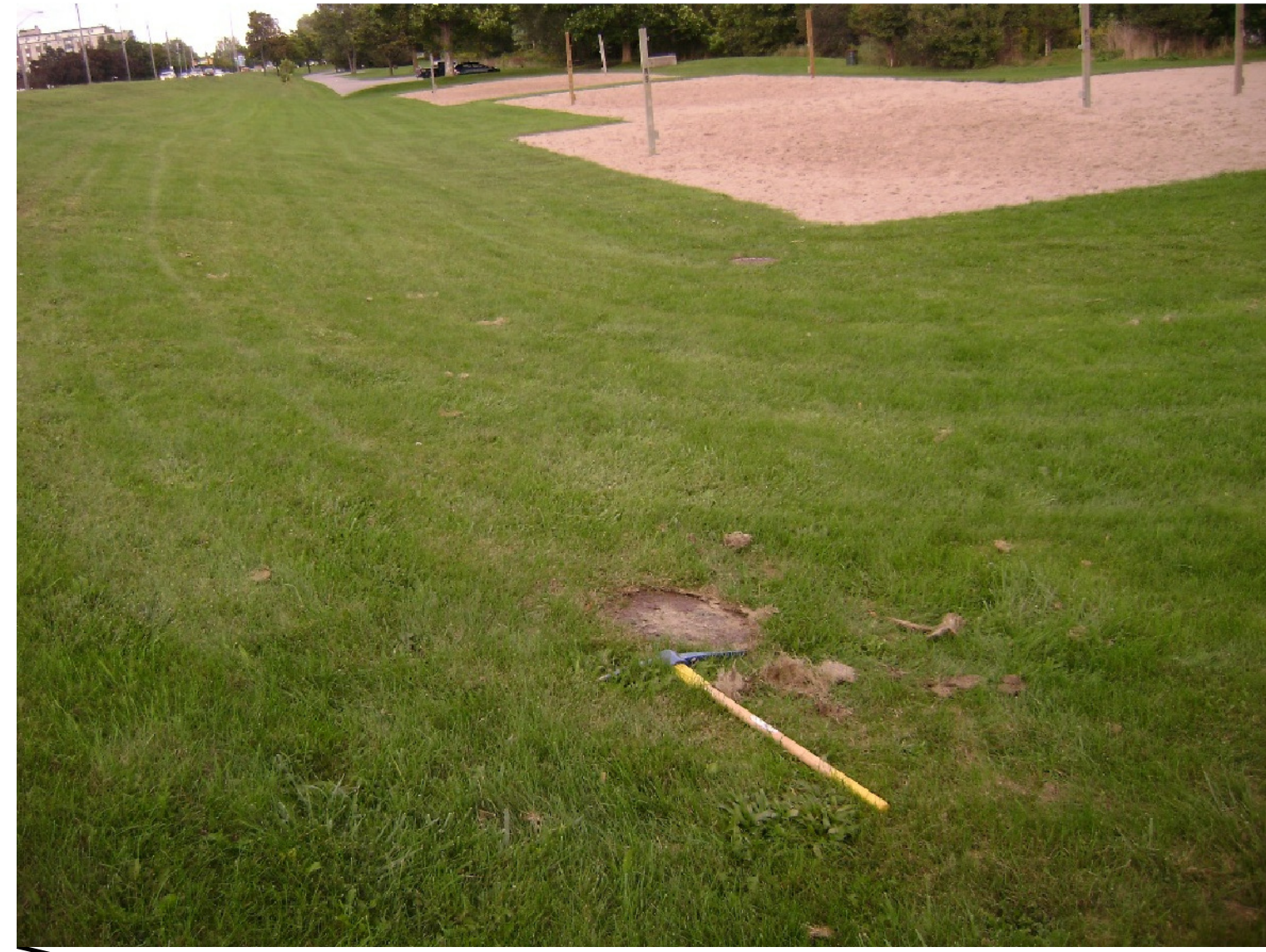
EXISTING YORK TRUNK SEWER ALIGNMENT ADJACENT TO VOLLEYBALL COURTS IN SILVERCREEK PARK
