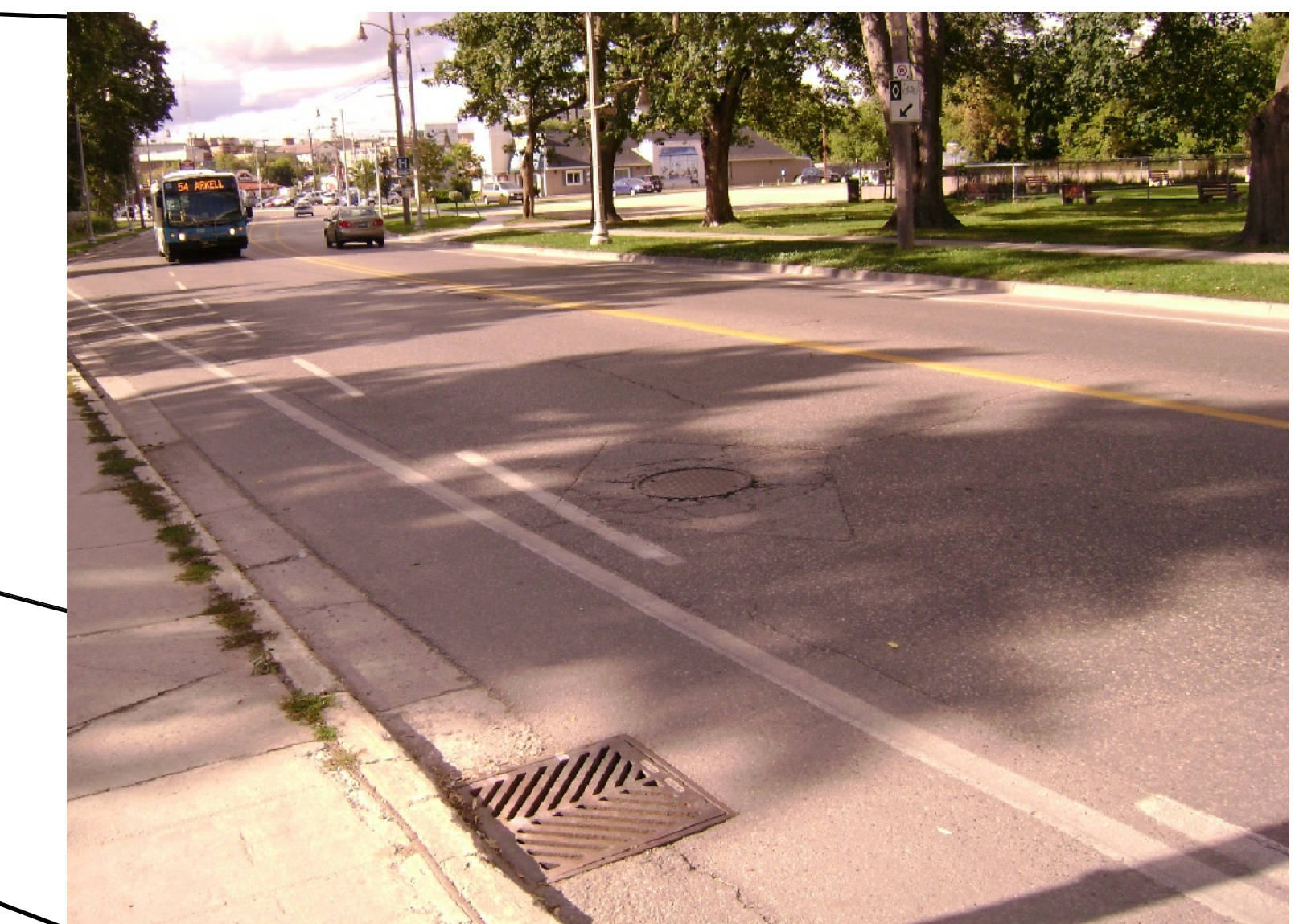
EXISTING YORK TRUNK SEWER ALIGNMENT AT GORDON STREET UNDERCROSSING
