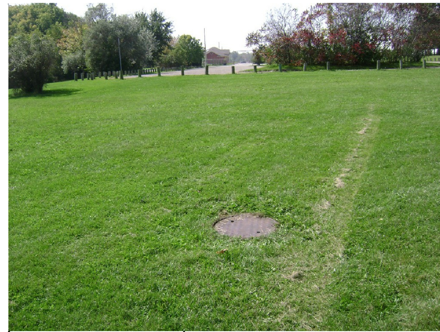
EXISTING YORK TRUNK SEWER ALIGNMENT LOCATED IN ERAMOSA RIVER PARK
