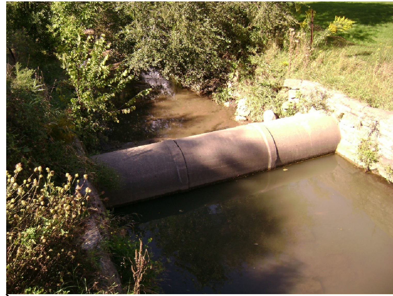
EXISTING YORK TRUNK SEWER CROSSING MUNICIPAL DRAIN IN SILVERCREEK PARK, BETWEEN EDINBURGH ROAD AND GORDON STREET
