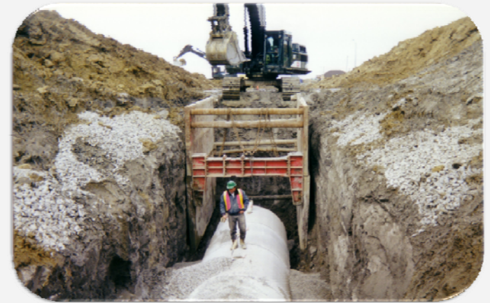
Typical Open-Cut Sewer Trench
