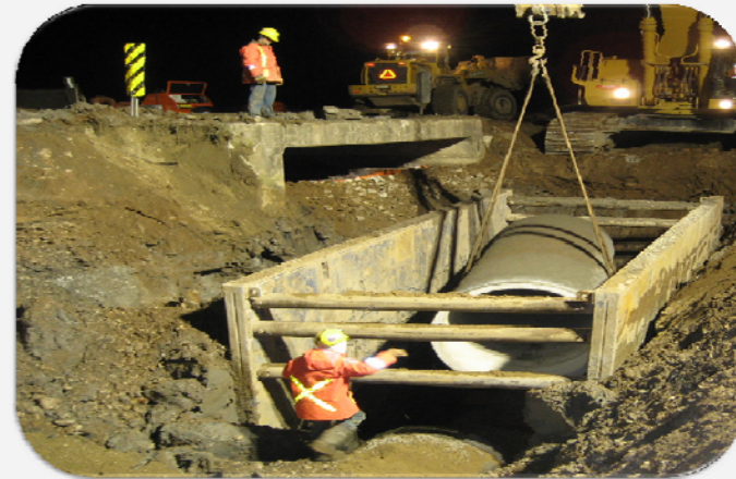
Use of a Trench Box
