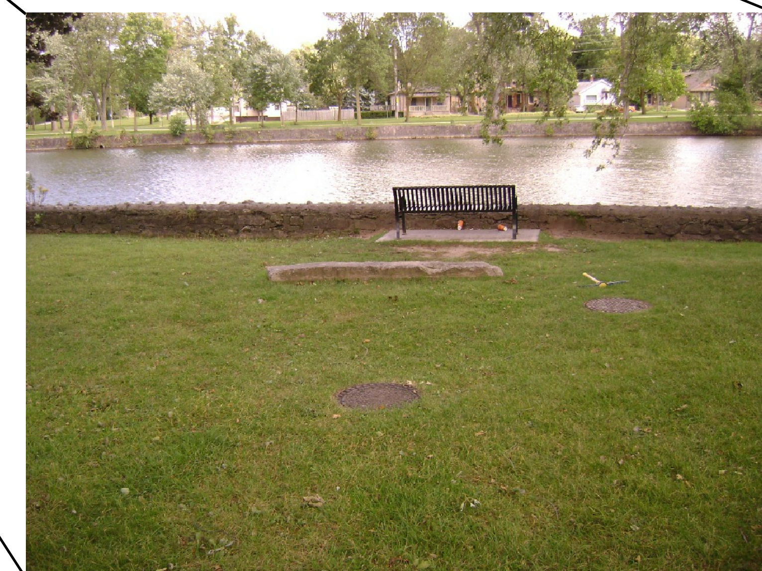
EXISTING YORK TRUNK SEWER ALIGNMENT IN SILVERCREEK PARK LOOKING SOUTH TOWARDS WATER STREET
