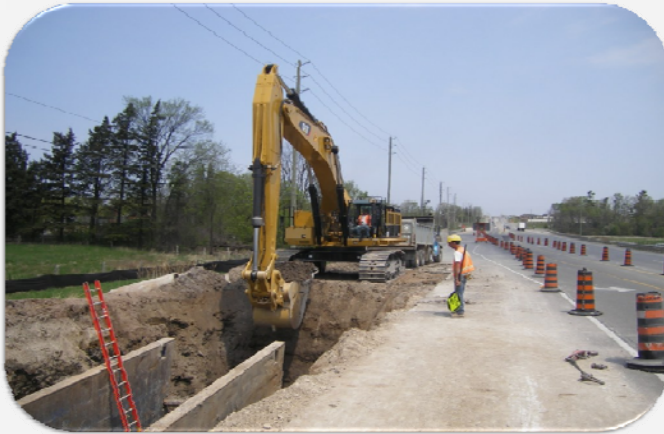
Open-Cut Sewer Construction on a Road Shoulder
