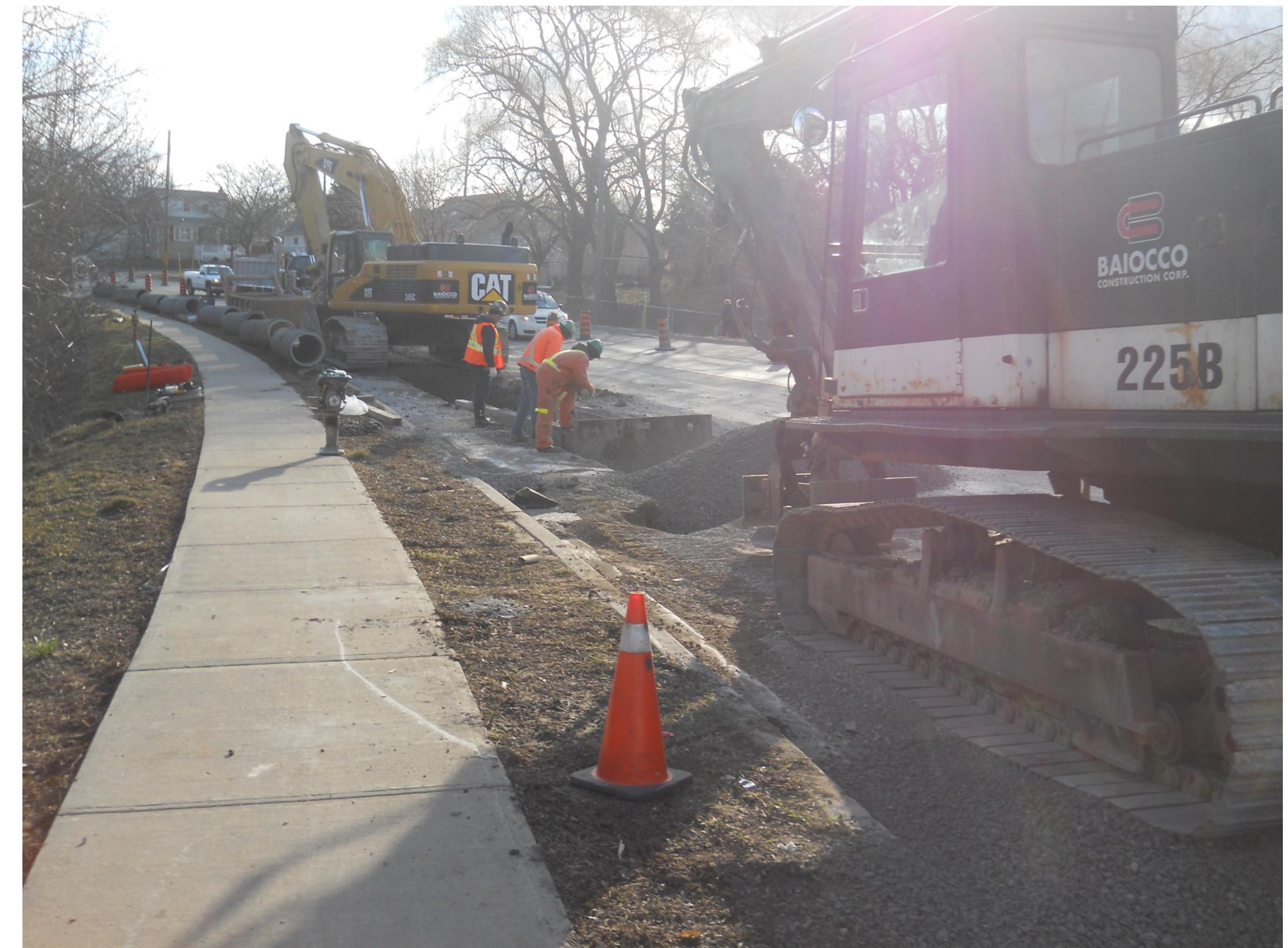
Open Cut Construction in St. Catharines
