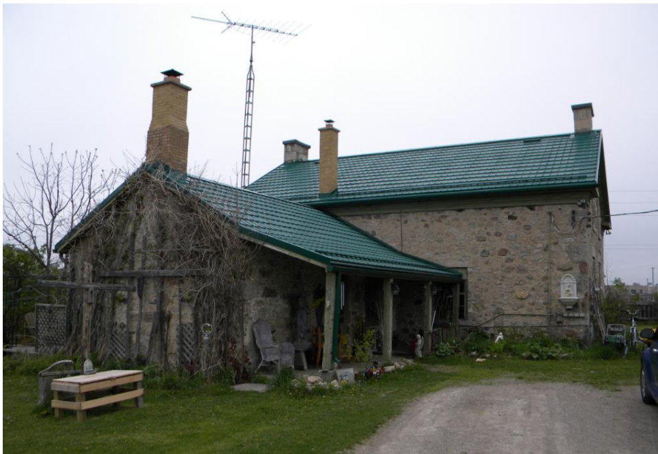
Figure 8 – Farmhouse tail, viewed from southeast. (Planning Services)
