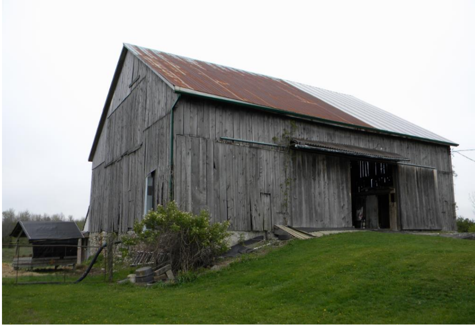
Figure 5 – Barn, viewed from north. (Planning Services)
