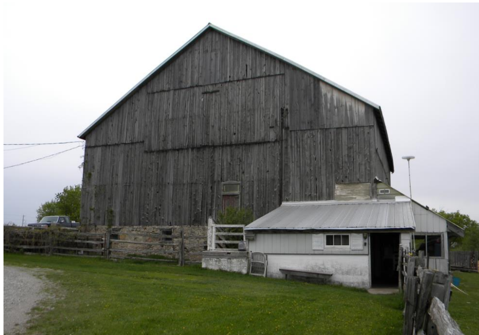
Figure 6 – Barn, viewed from west. (Planning Services)
